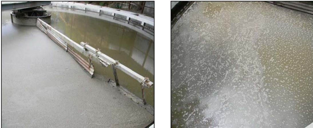
Fig. 25: A View of Secondary Clarifier
