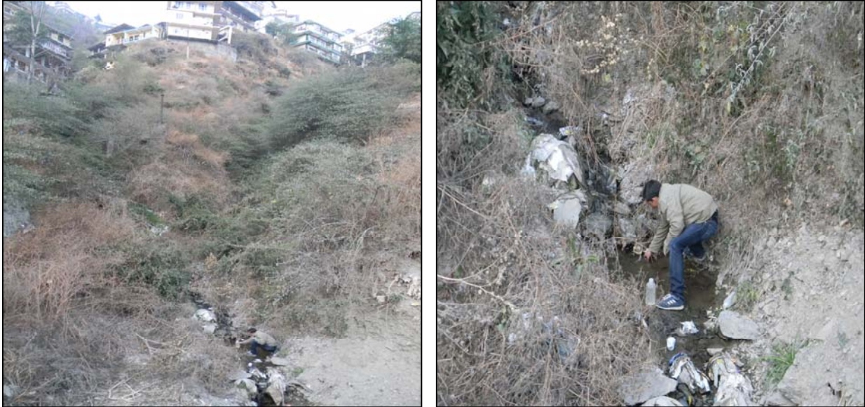
Fig. 21: A View of Sanan Open Drain in Study Area
