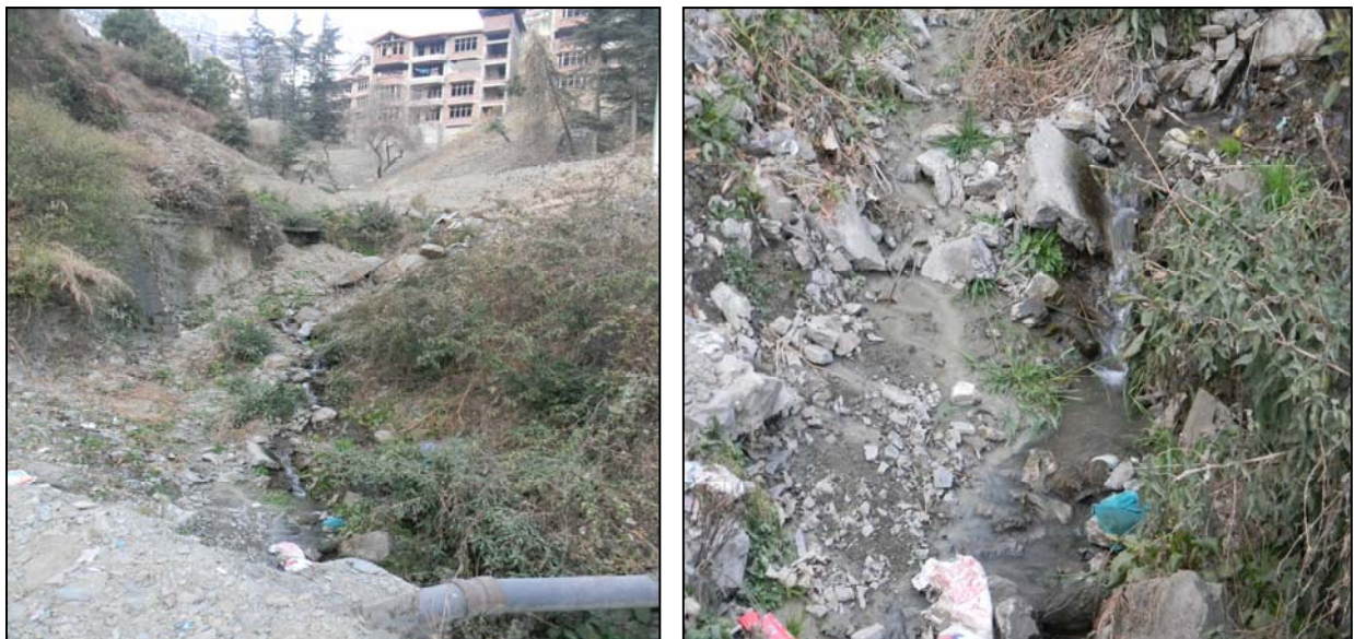
Fig. 20: A View of Housing Board Colony Open Drain
