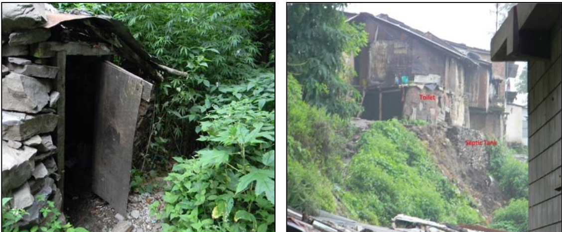
Fig. 28: Open Defecation and Septic Tanks in the Study Area
